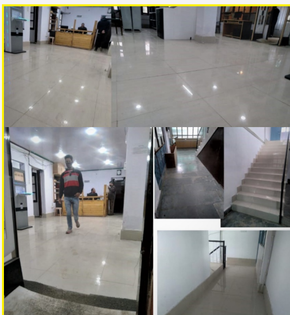
Tiling of Central Library
